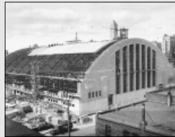
The Minneapolis Armory, shown here during construction in 1935.
