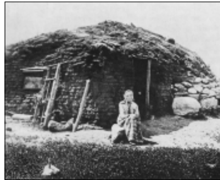
Early settlers built sod houses such as this when timber was scarce. Pieces of sod were stacked similarly to bricks, and were sometimes fastened together with a mortar of clay and buffalo grass.
