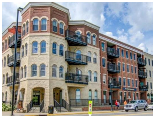
Figure 10: New Multifamily Development in Downtown Stillwater, MN
