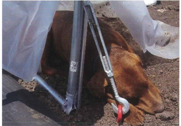
*Photo 3. We modified the earth anchor system to make the mobile modular hoop house sturdier. Note how soundly Kodiak is sleeping, confident that it won't blow away again.*
