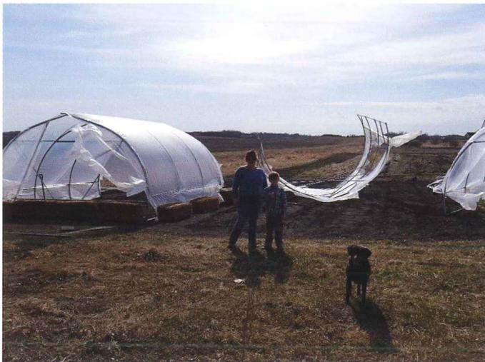
*Photo 2. Big winds can mean disaster. After this catastrophe, we modified our anchoring system.*
