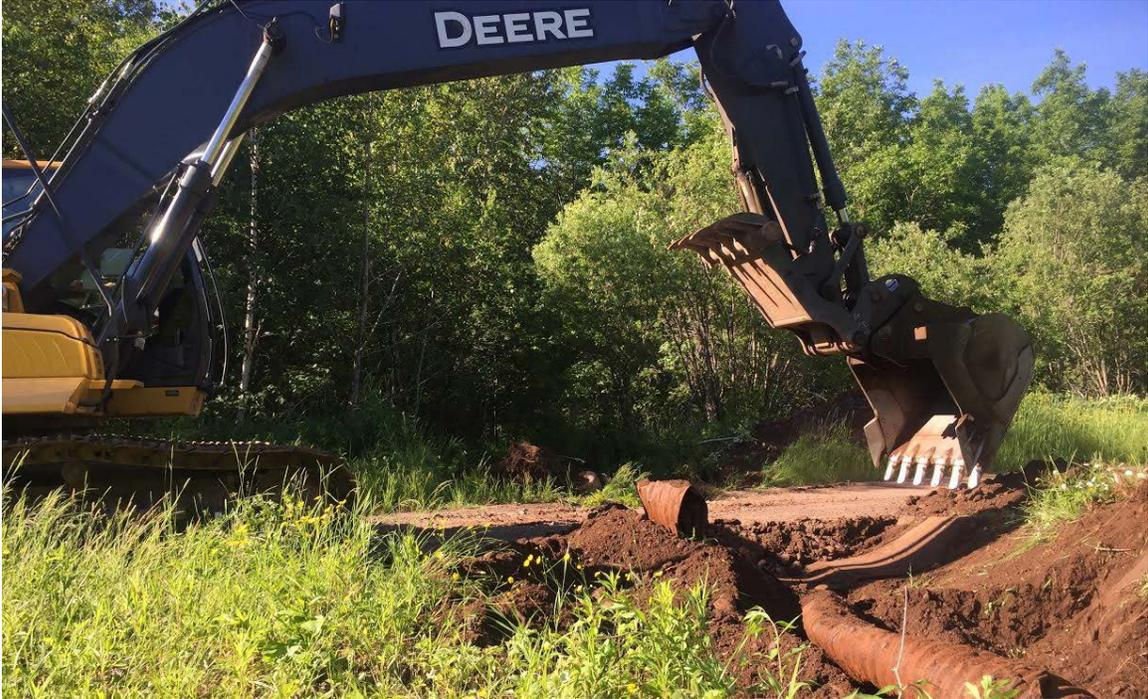
**Figure 43.** Replacing old culvert at Defrense Road.
