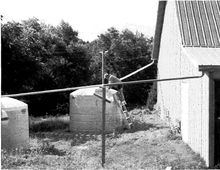
**Rainwater storage tanks with the gutter system coming off the 40' x 50' barn.**
