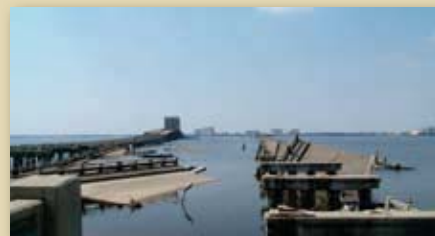
Hurricane Katrina damage to bridge
