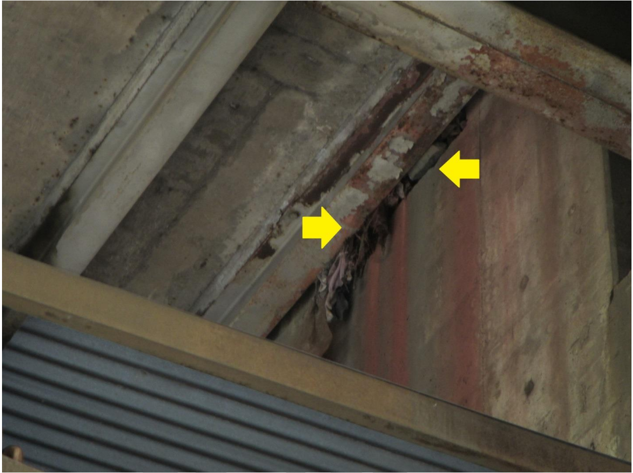
Figure 6. A possible crevice that houses bats near the coarse crusher. The yellow arrows point to the large crevice.
