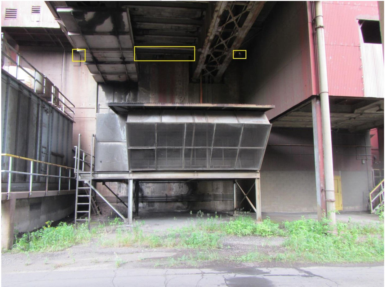
Figure 5. Possible roost structures near the coarse crusher. Areas outlined in yellow are suspected areas of bat emergence, though any crevices that may house bats are unable to be seen from the ground.
