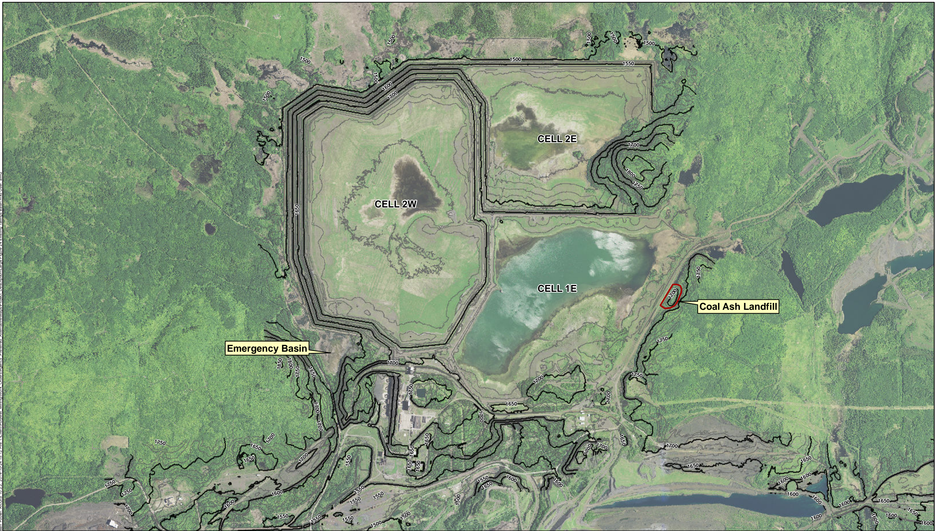
Large Figure 24 EXISTING TAILINGS BASIN NorthMet Project Poly Met Mining Inc. Hoyt Lakes, MN
