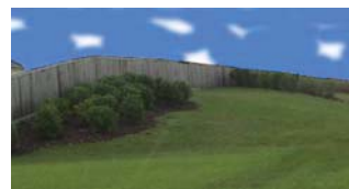
Combination of earth berm and noise wall
