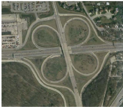
CLOVERLEAF INTERCHANGE RAMP
