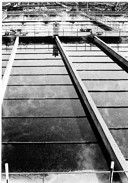
The settling tanks at the Metro Plant, the primary phase of the wastewater treatment process.
