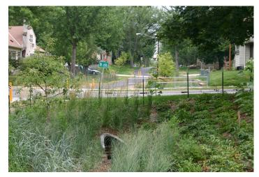
Minneapolis removed a 5 ½ block section of road to create a green way that provides treatment of stormwater prior to discharge into Crystal Lake.
