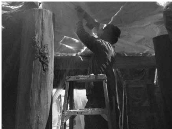
Construction of the walk-through Iron Range mine inside “Then Now Wow”
