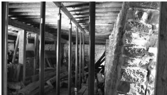
Veblen Farmstead hay barn stabilization
