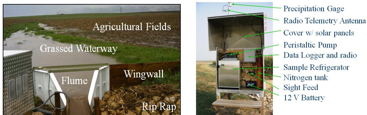
Figure 1. Flume-wing-wall installations at Pioneer Farm.
