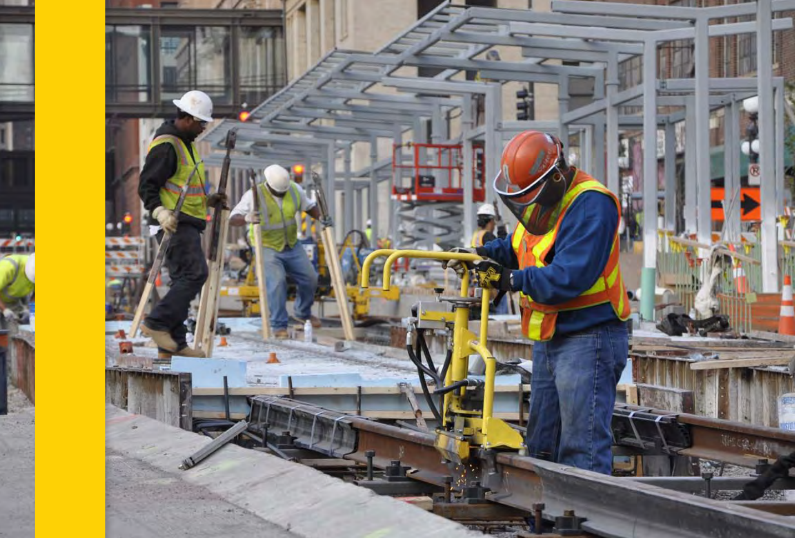
A construction worker grinds rail to remove irregularities at the Union Depot station in downtown St. Paul.
