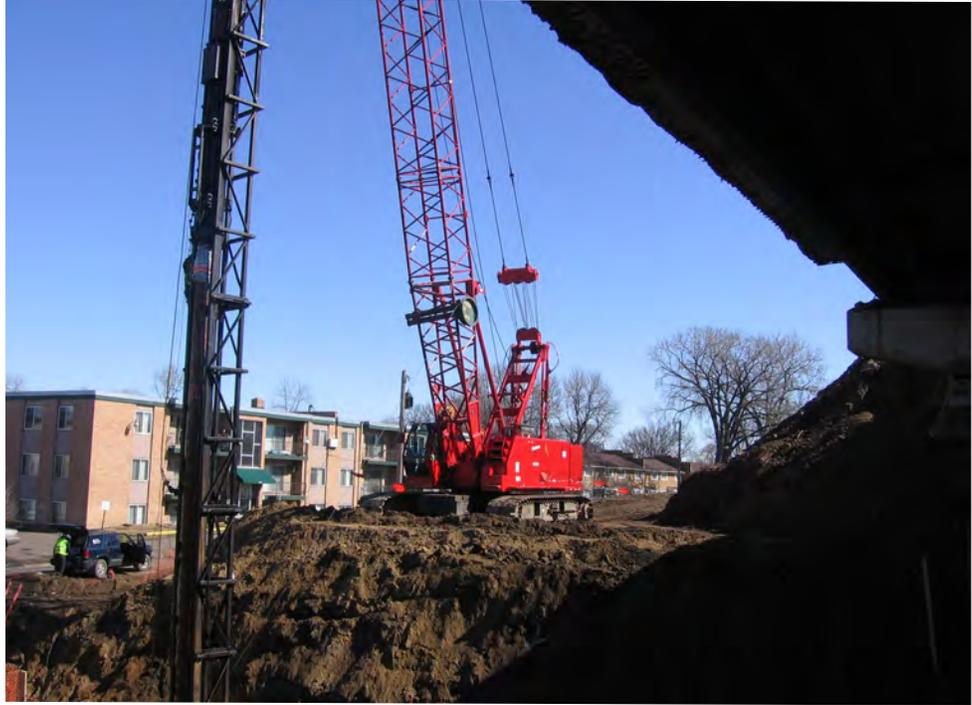
Construction crews need to drive piles deep enough to provide support for a bridge while not overdriving, which wastes resources.
