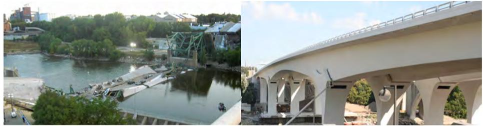
The collapse of the I-35W bridge (left) in August 2007 intensified the interest in bridge health monitoring. In this project, researchers helped Mn/DOT staff evaluate the instrumentation proposed for monitoring the new St. Anthony Falls Bridge (right), which opened in September 2008.
