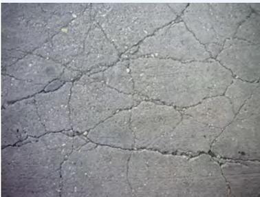
Cracks on concrete decks are a leading cause of bridge deterioration.
