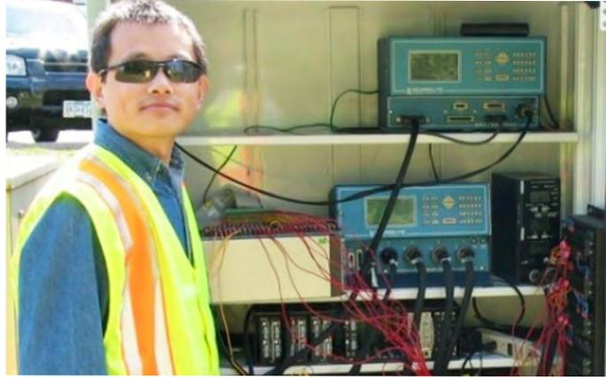
SMART-SIGNAL's data collection devices installed in a France Avenue signal controller cabinet received data from vehicle detection units and the traffic signal controller.
