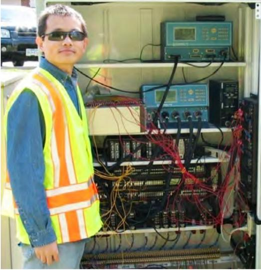
**University of Minnesota researchers developed the SMART-SIGNAL system to cost-effectively collect and archive high-resolution traffic signal data and automatically generate real-time performance measures such as travel time, queue length and intersection delay. Engineers can use SMART-SIGNAL data, collected via detection units installed in signal cabinets like this one, to optimize timing schedules on each traffic signal to reduce congestion without additional road construction.**
