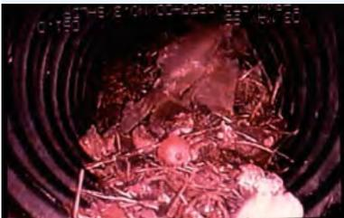
Rodent nests within the drainage pipe are one of the more common maintenance problems for subsurface drainage systems.
