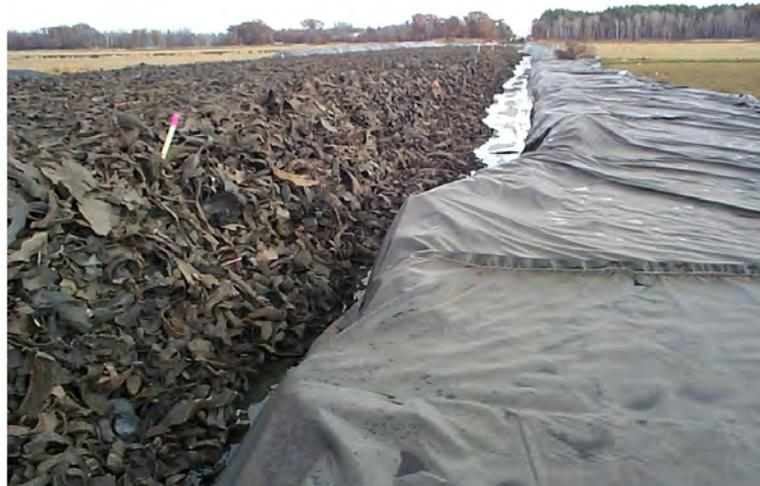
Shredded tires were placed within a layer of geotextile permeable fabric and enclosed in “burrito wrap” fashion to form the new road base. This wrap was used to keep the tire material from migrating into the soft undersoils.
