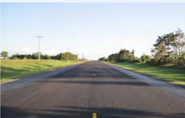
Chip seals are typically applied to HMA pavements that are four to seven years old and can make these pavements look like new.
