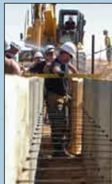
(top) From a hilltop on the U.S.-Mexico border, Spc. Michael Elmer spots four people on foot moving toward the fence below. (left) 133rd Airlift Wing Civil Engineer Tech. Sgt. Kurt Huver checks the level on the concrete forms for a fence along the U.S.-Mexico border near San Luis, Ariz.
