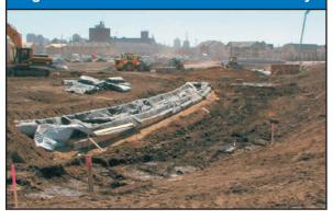
**Level Spreaders:** Level spreaders are located upslope from filtration basins at the transition point between short grass prairie and wetland community to promote even, low-velocity sheet flow into the filtration basins, preventing erosion and enhancing filtration.
