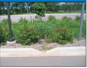
Adjacent to the runoff model is a parking lot with swaled rain gardens. The swales have 2 feet of sand topped with 6 inches of sandy top soil and planted with drought resistant (mostly native) plants. A subsurface drain below the sand and overflow yard-drains help manage excessive rain events. The overflow and subsurface drains go directly to a NURP pond.
